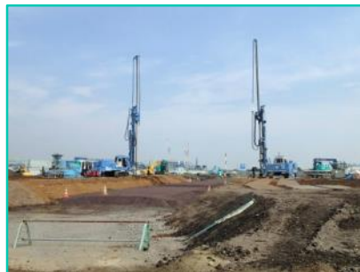
Haneda Airport land infrastructure development construction (Foundation improvement)
