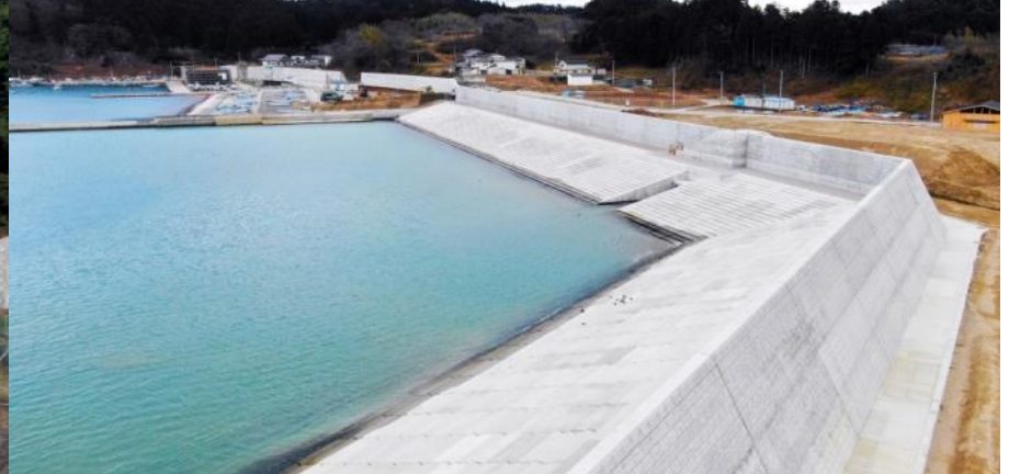
Mutsugaura Fishing Port seaside disaster recovery construction (Iwate Prefecture)
