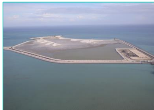
Nakagusuku Bay Port sediment disposal zone embankment construction
