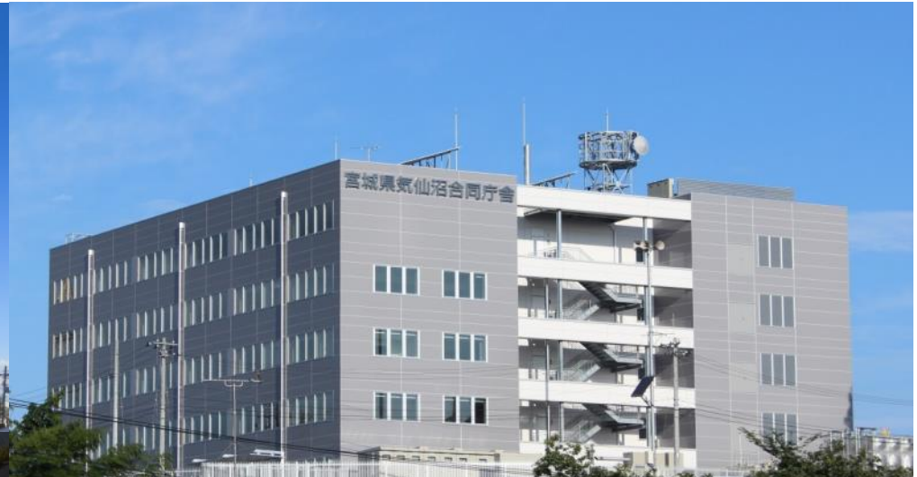
New building construction for the Kesenuma government office complex (Miyagi Prefecture)
