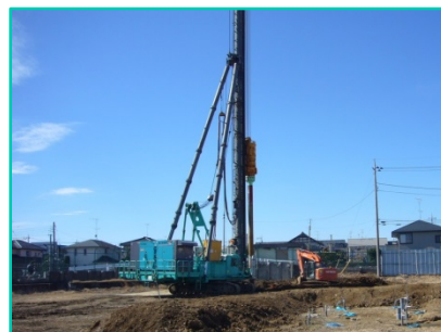
東松山土壌改良工事 (ground improvement)
